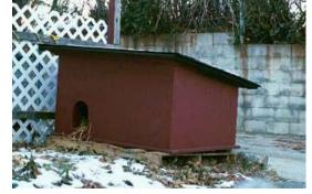
This insulated cat house has a great design feature in that the shingled roof is hinged to allow easy access to the interior for maintenance. Pros: Sturdy design, large enough to house multiple cats, provides protection from predators. Cons: Building requires some degree of skill. Supplies cost are medium compared to other designs.
